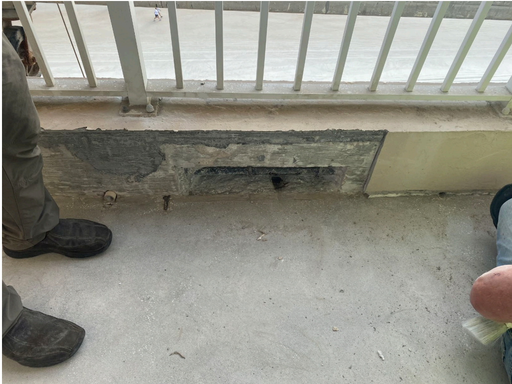
Picture 2: Unit 701 concrete repair
