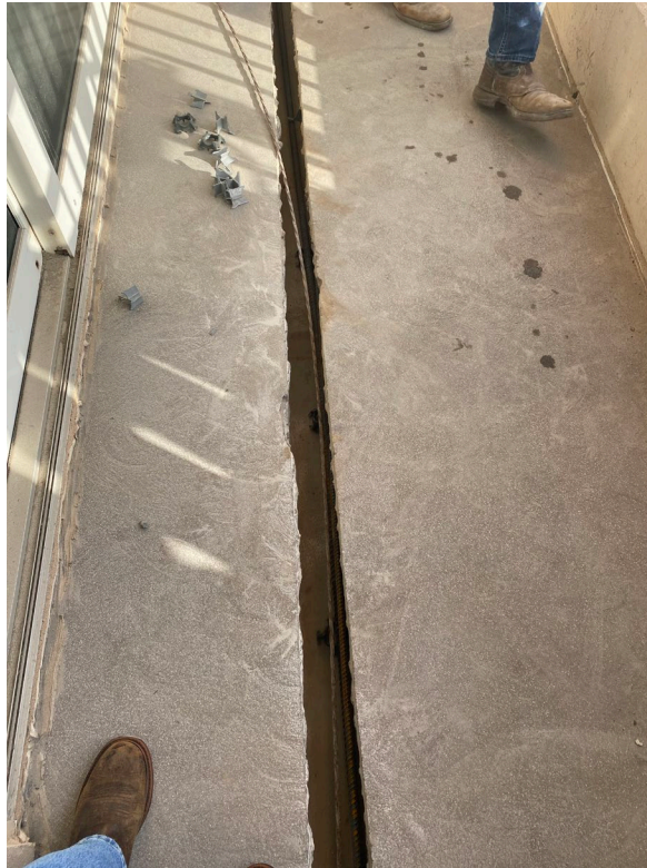
Picture 1: Unit 202 concrete repair
