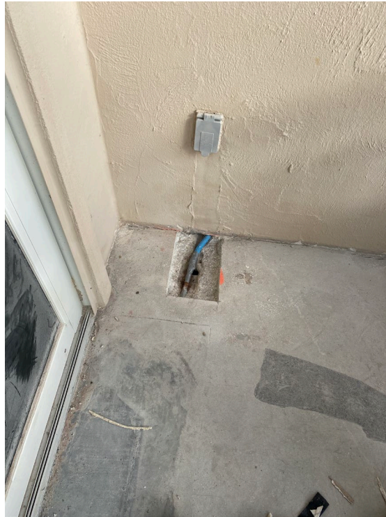
Picture 3: Unit 701 concrete repair
